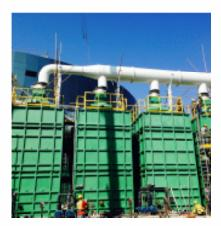
With a countless range of structured and random packed medias to suit the specifics of even the most challenging of municipal or industrial problems, Mytilus biotrickling filters are used around the world. BIOREM offers state-of-the-art modular standard systems as well as fully customized rectangular, cylindrical or field-erected systems.
